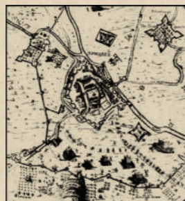
The Newark defences. Some of the earthworks remain intact to this day.
